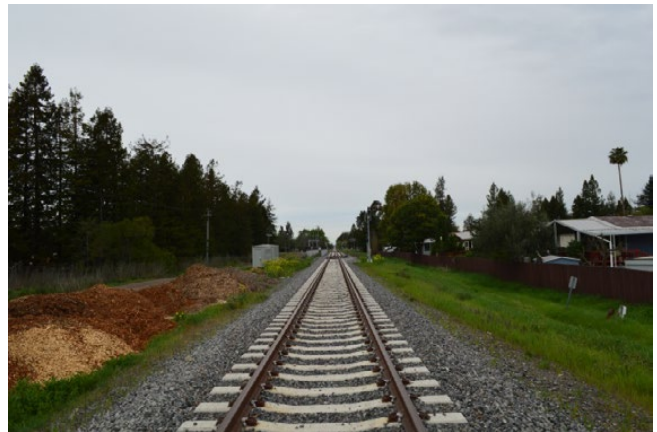
Site Photo 4 —Northwest Pacific Railroad
